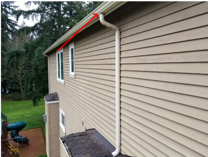
Downspout appears to be clogged and full of water.
