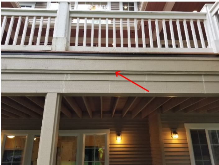
The water coming through the trim is causing the paint to run.
