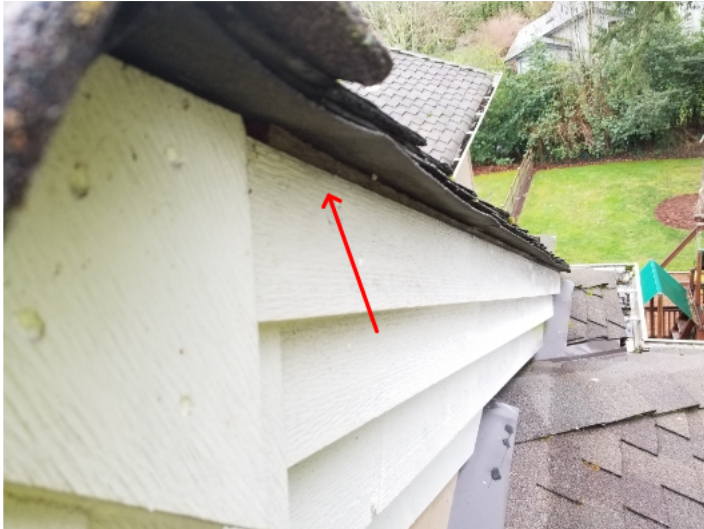
Missing kick out flashing.
