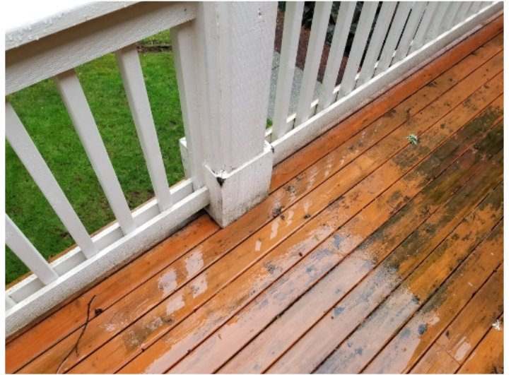
Missing paint and some of the wood is starting to deteriorate.
