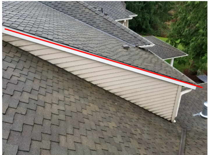
Missing rake flashings.
