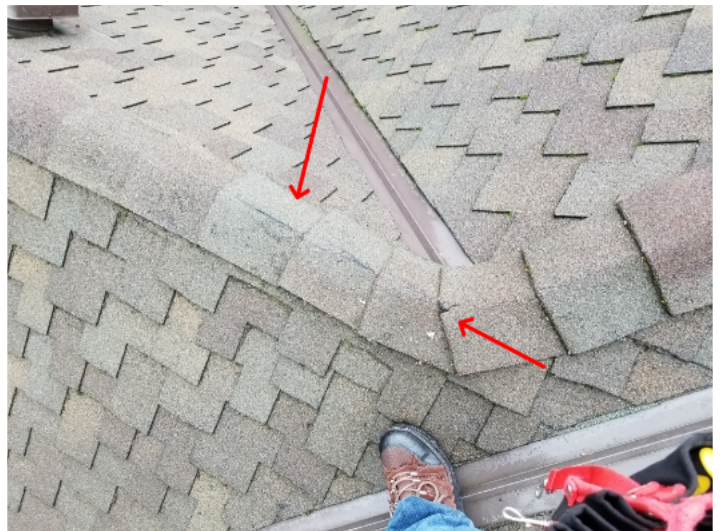
Damaged ridge cap.
