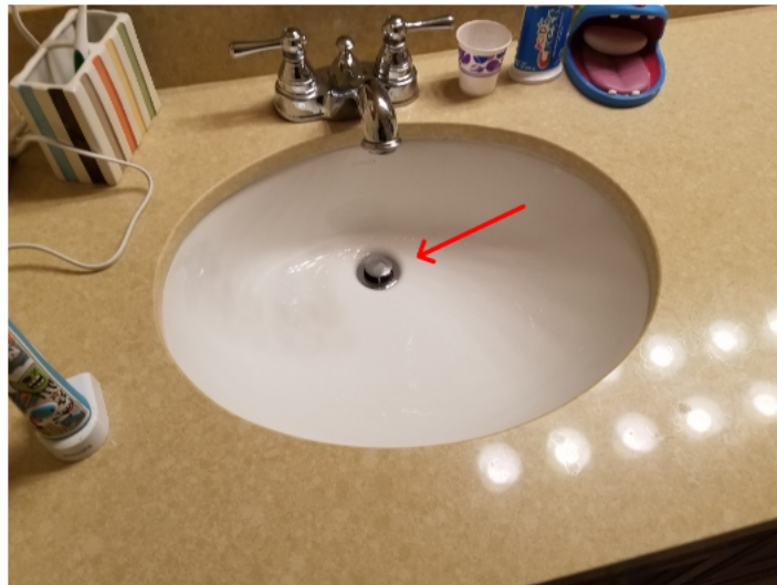
stoppers do not function properly.
