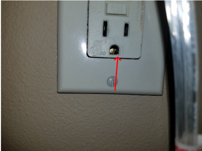
broken prong stuck inside
