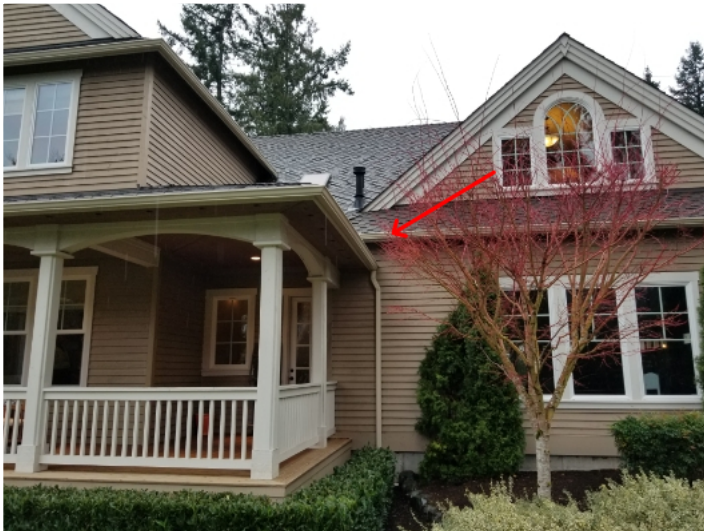
Missing kick out flashing.
