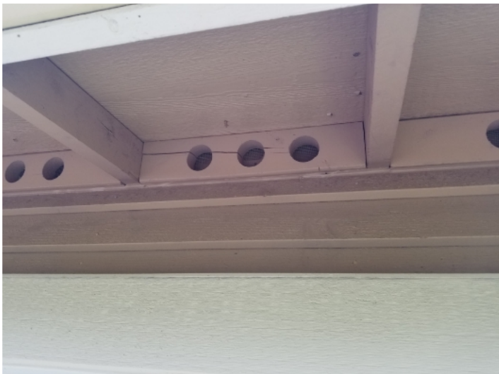
Cracked bird block.
