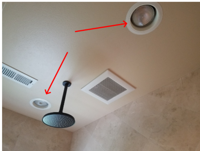
improper wet area light fixtures
