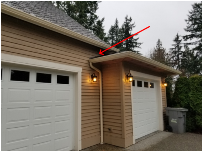
Missing kick out flashing
