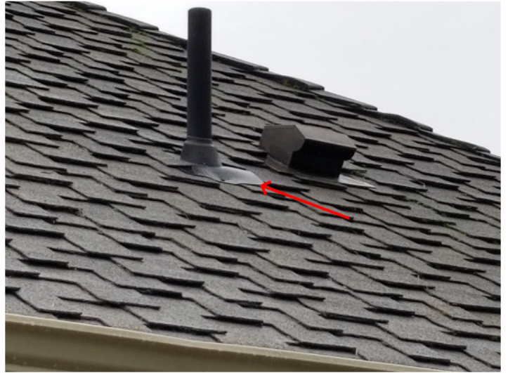
Puckered plumbing boot.
