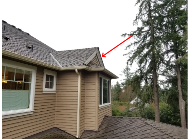
Missing rake flashing and exposed plywood.
