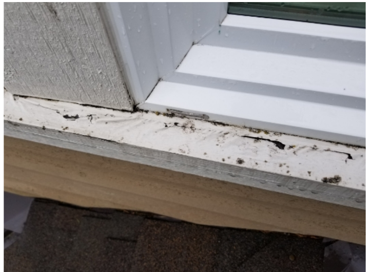
Missing paint and some of the wood is starting to deteriorate.
